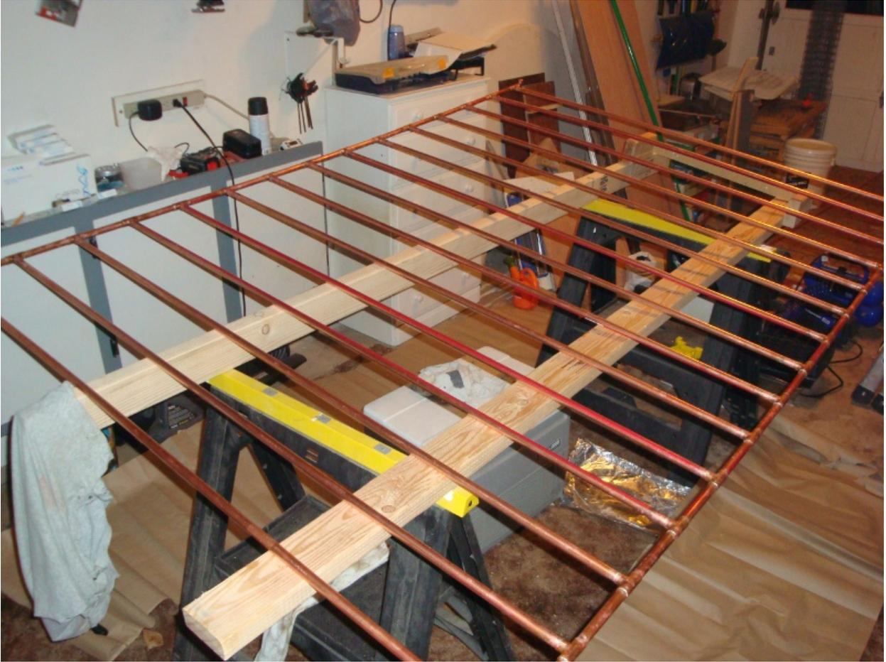
Then we installed the copper grid into the insulated collector box. It's tilted slightly, which is to allow the water to drain out.
