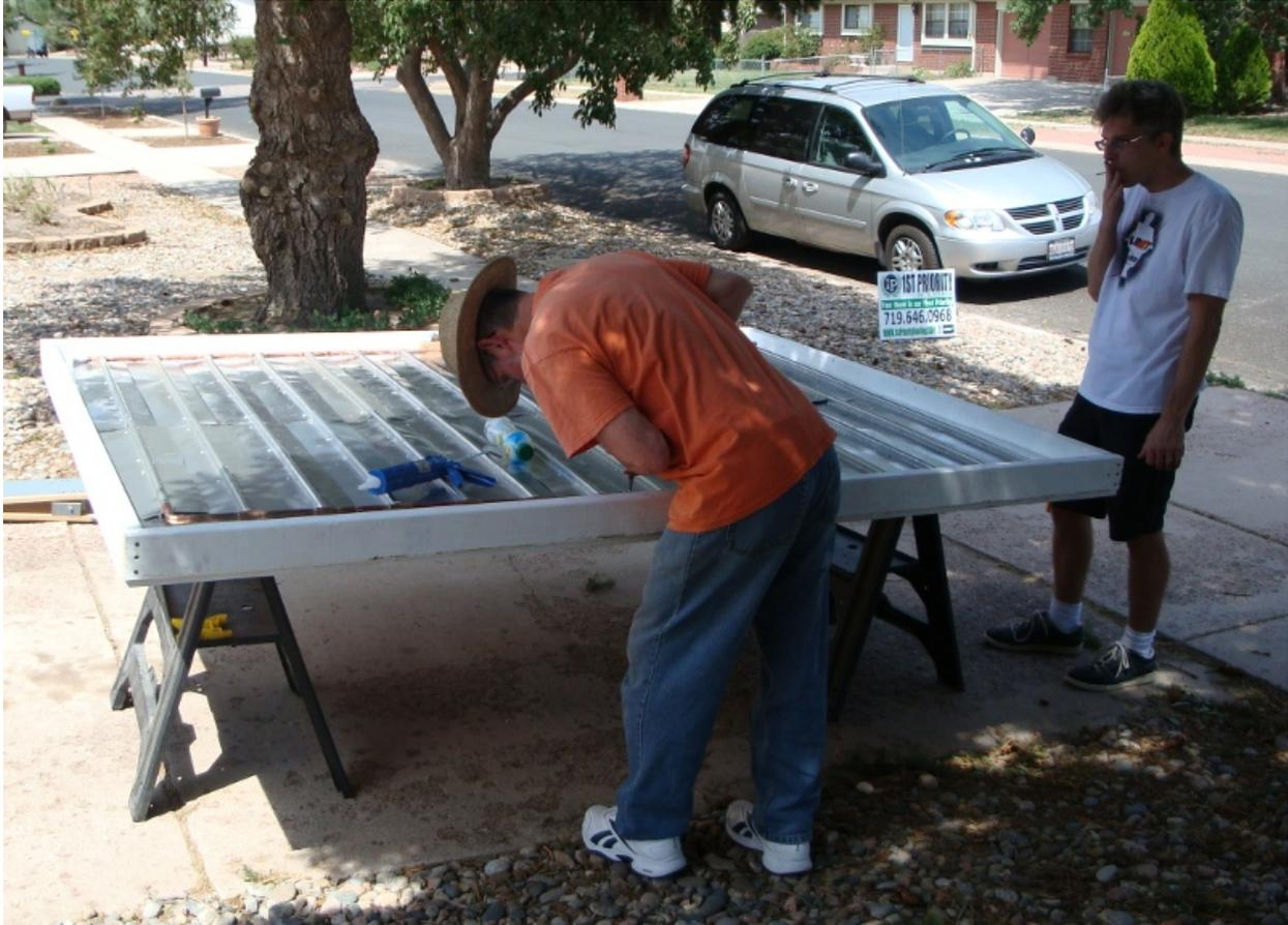
And then some corrugated polycarbonate glazing on the front, attached with short hex-head screws with rubber gaskets. I drilled the holes in the poly considerably larger than the screws, since it'll want to expand and contract (and I don't want it to crack). Of course, liberal use of silicone here too.
