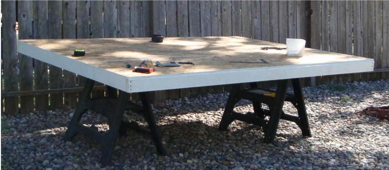
We painted all of the pieces with 1-2-3 primer, and assembled it using a bunch of miscellaneous 2" screws I had lying around. To ensure an airtight seal, we put a bead of silicone along all edges to be joined. Inside the box, we put a 1" layer of foil-backed polyisocyanurate insulation; this should reduce the amount of heat lost out the back of the collector.
