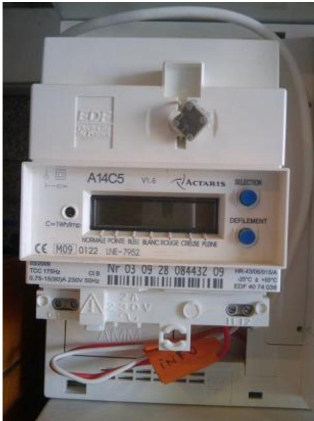
Open the bottom part (be careful, if there is a metallic security to prevent opening, you may be looking for the wrong thing!!) of the electric meter. On the right, you should see I1 and I2 : it is there you should plug the teleinfo modem. On this photo, there are both a teleinfo modem and a heating programmer plugged:
